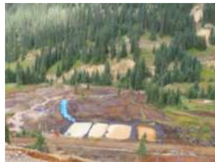
Figure 3: Settling ponds built near Gold King mine allow acid mine drainage to pool, where contaminants can settle to the bottom and acidity can be treated. (US EPA via Flickr, 2015).
